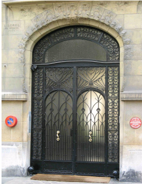
Main door of the building.
