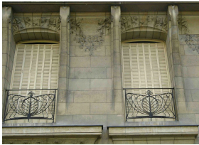
Detail of the first floor.
