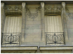
Detail of the first floor.
