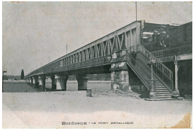
The Passerelle Eiffel crossing the Garonne river in Bordeaux, 1858-1860.
