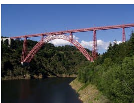
The Viaduct of Garabit in Cantal. Technical feat of Gustave Eiffel in 1884.
