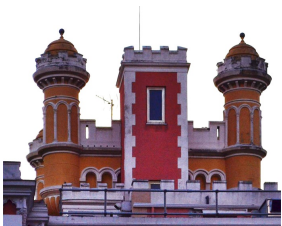
Castellated towers, château des Ollières.
