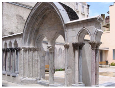
Saint-Jean Cloister in Bagnères-de-Bigorre, 13th century, columns made out of red griotte marble
