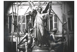
Thanks to the advanced patents of the technique of electroplating, Christofle realizes the monumental groups on the top of Paris Opera facade. Group of Poetry.
