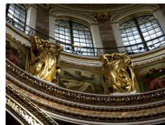
Dome of Saint Isaac's Cathedral in Saint Petersburg. The angels statues (6 meters high) were made in electroplating. ca 1858
