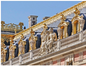
Palace of Versailles, decor of the marble courtyard. The roofs of the Palace of Versailles were gilded with mercury under Louis XIV.
