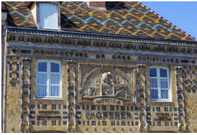
Front of former Gréber manufacturing workshop in Beauvais.
